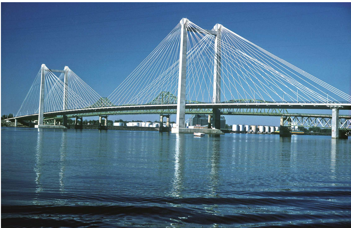
Figure 27: Pasco-Kennewick Bridge, 1978, 299 m
