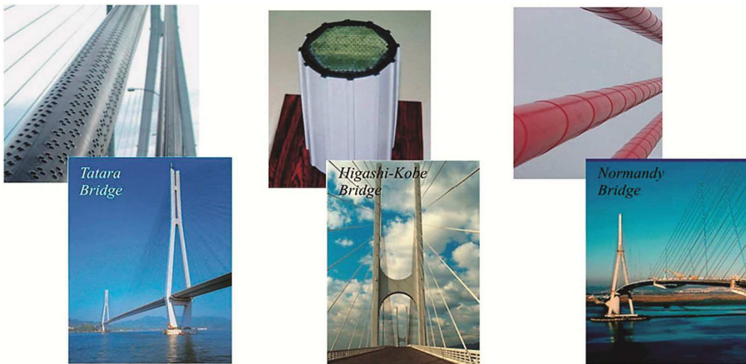
Fig. 71: Some well-known applications of surface profiling
