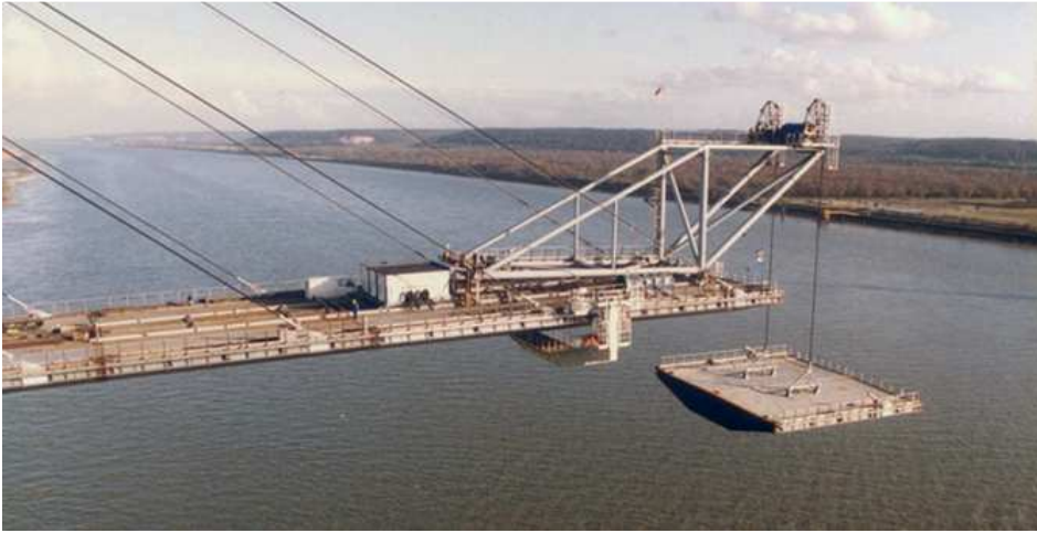
Figure 57: Lifting of beam section
