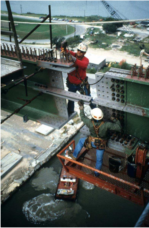
Figure 39: Joining the main girders with high-strength bolts
