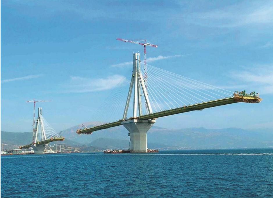
Figure 67: Free cantilevering
