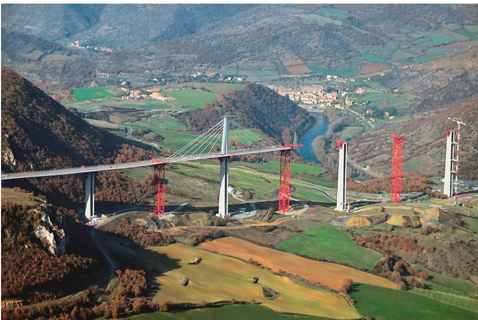
Figure 69: Further launching
