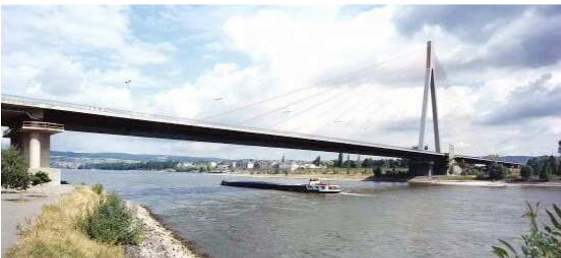
Figure 24: Neuwied Bridge, 1978, 235 m and 212 m
