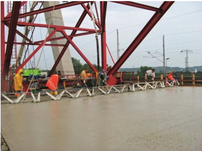
Figure 47: Planing of roadway slab
