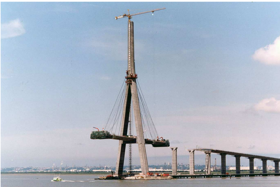
Figure 56: Free - cantilevering
