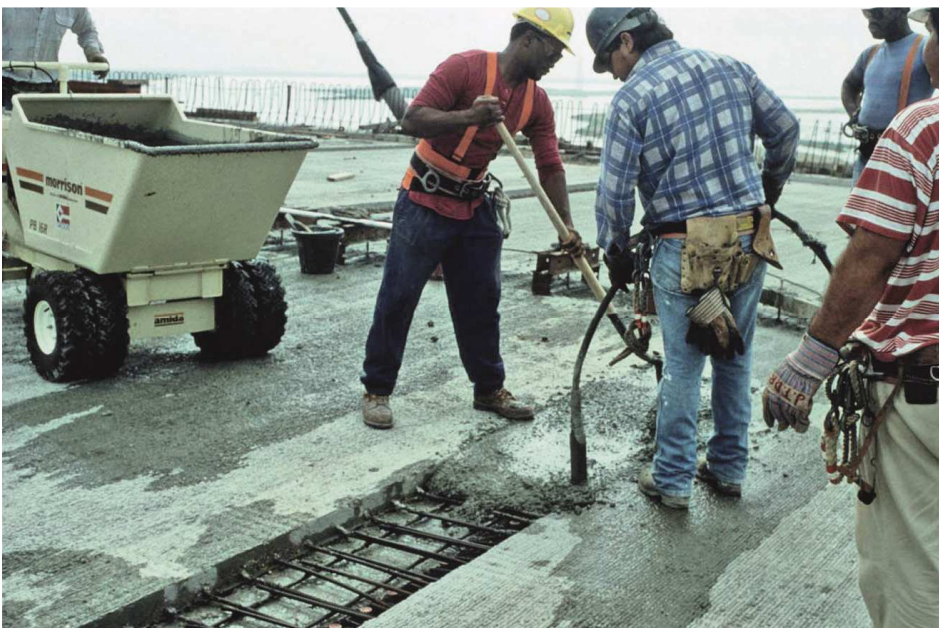
Figure 41: Casting of joints
