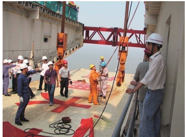
Figure 62: Fitting of the final beam element
