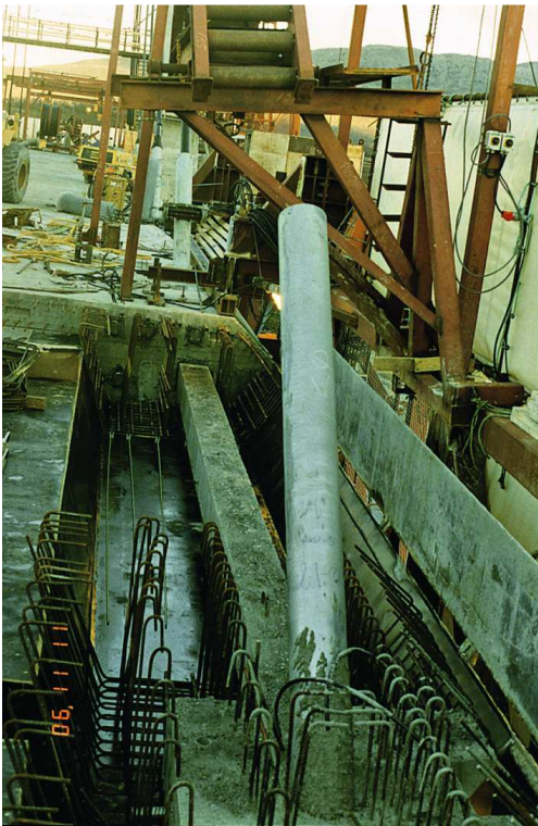
Figure 32: Precast element in Form
