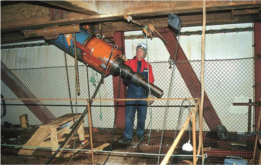
Figure 9: Stressing of a stay cable
