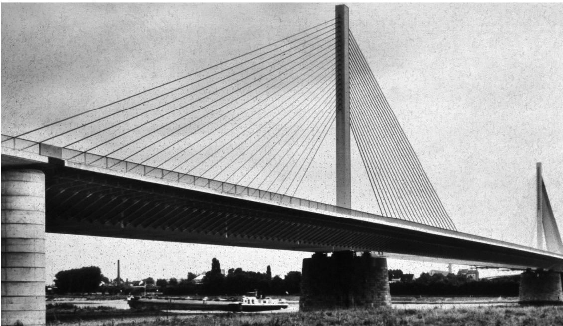
Figure 21: Bonn North Bridge, 1967, 280 m
