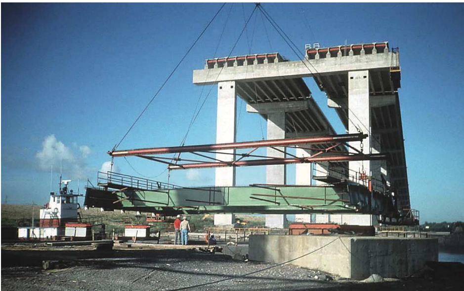
Figure 38: Lifting of girder grid from barge
