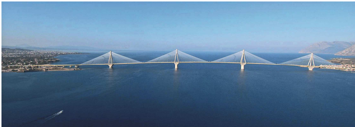
Figure 66: Rion Antirion Bridge, 2004, 3 x 560 m
