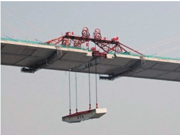
Figure 61: Lifting of the final section
