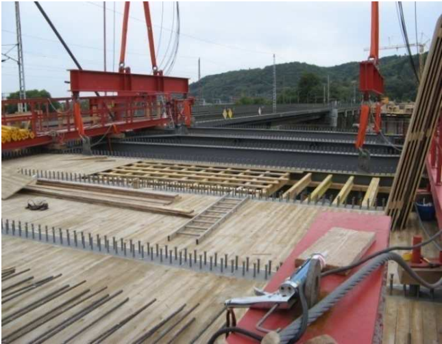
Figure 45: Falsework for roadway
