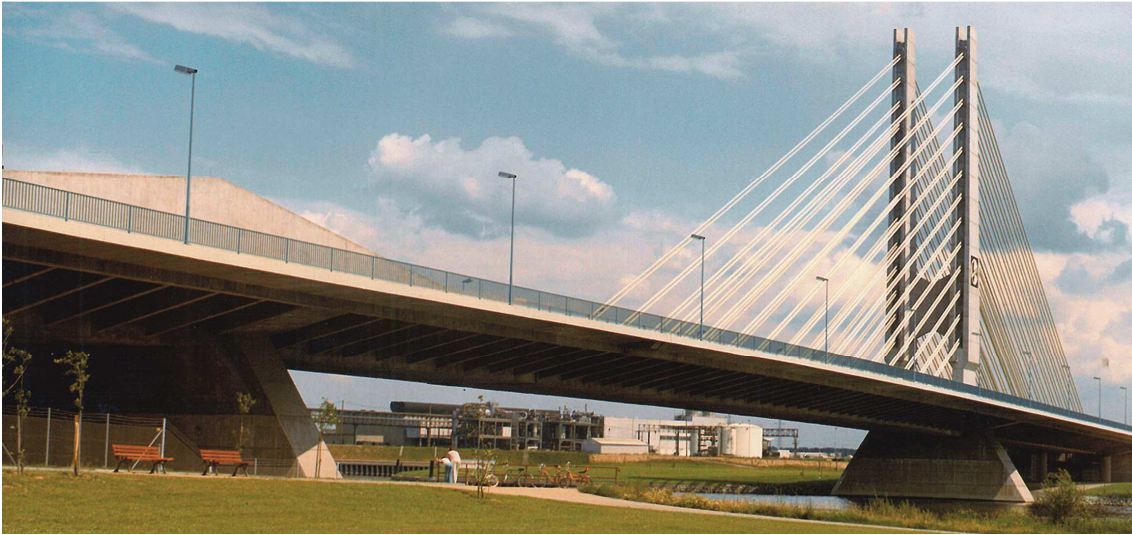
Figure 26: Main River Bridge at Hoechst 1972, 148 m
