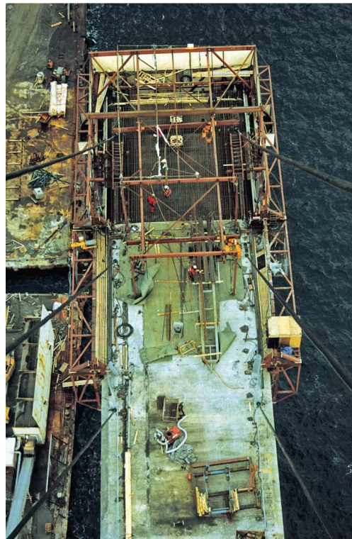
Figure 33: Traveler with final stay cables
