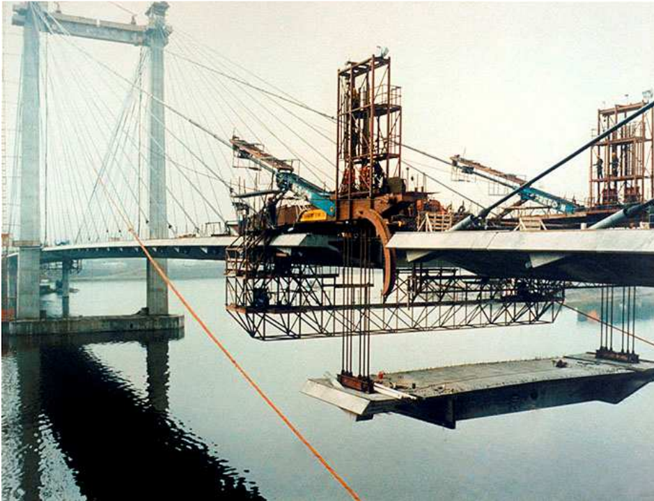
Figure 28: Lifting of the last precast element
