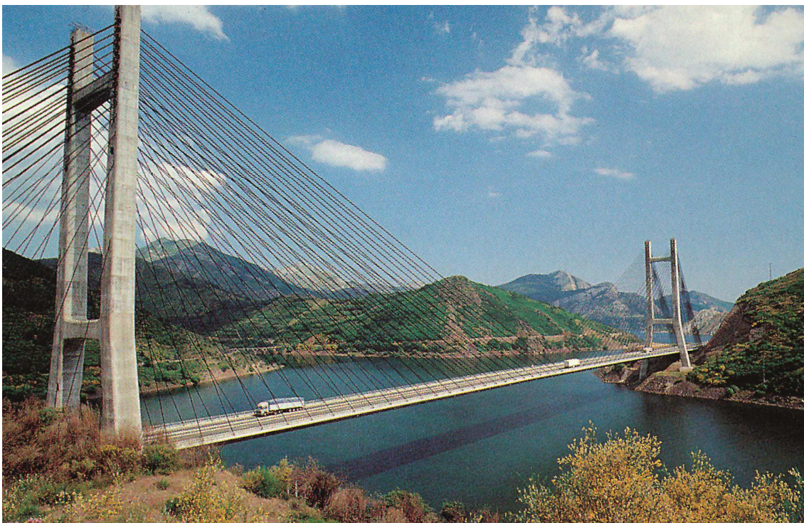
Figure 50: Barrios de Luna Bridge, 1984, 440 m
