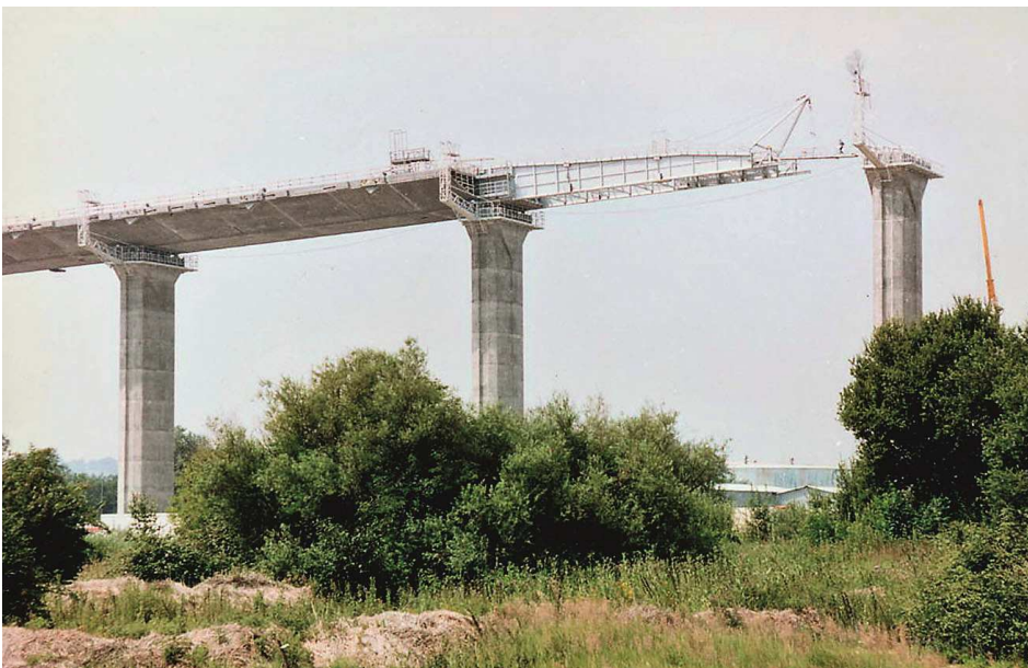
Figure 55: Launching nose
