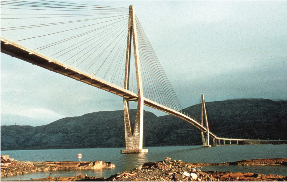
Figure 29: Helgeland Bridge, 1991, 425 m
