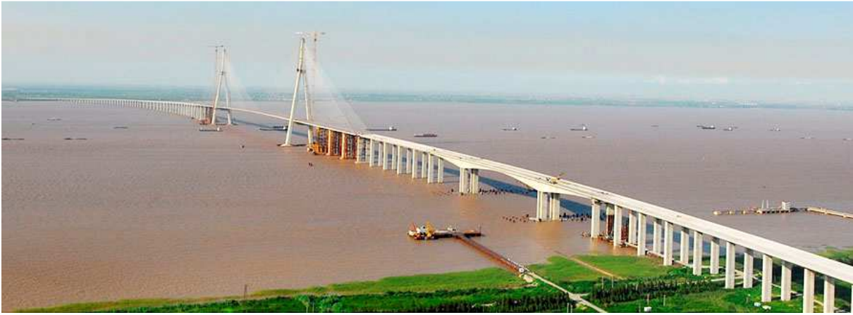
Figure 60: Sutong Bridge, 2008, 1088 m
