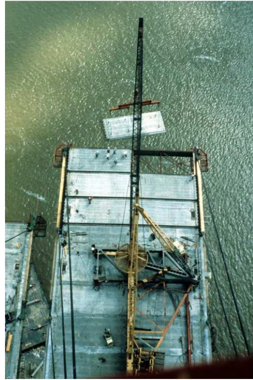
Figure 40: Lifting of precast slabs onto girder grid
