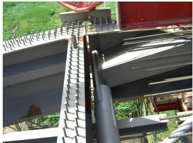
Figure 44: Aligning new section
