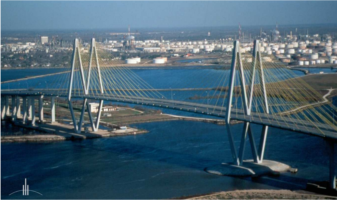
Figure 37: Baytown Bridge, 1995, 366 m
