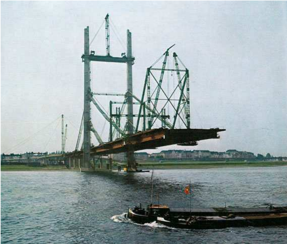
Figure 16: Free-cantilevering
