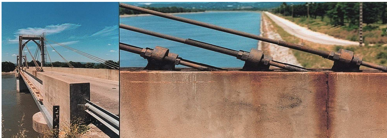
Figure 25: Donziere Bridge, 1952, 78 m
