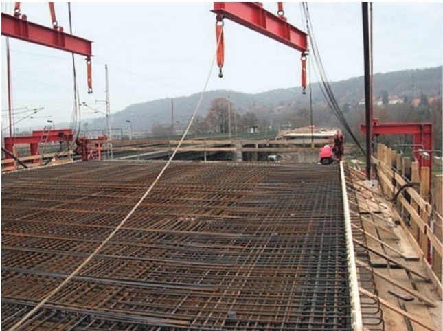
Figure 46: Reinforcement
