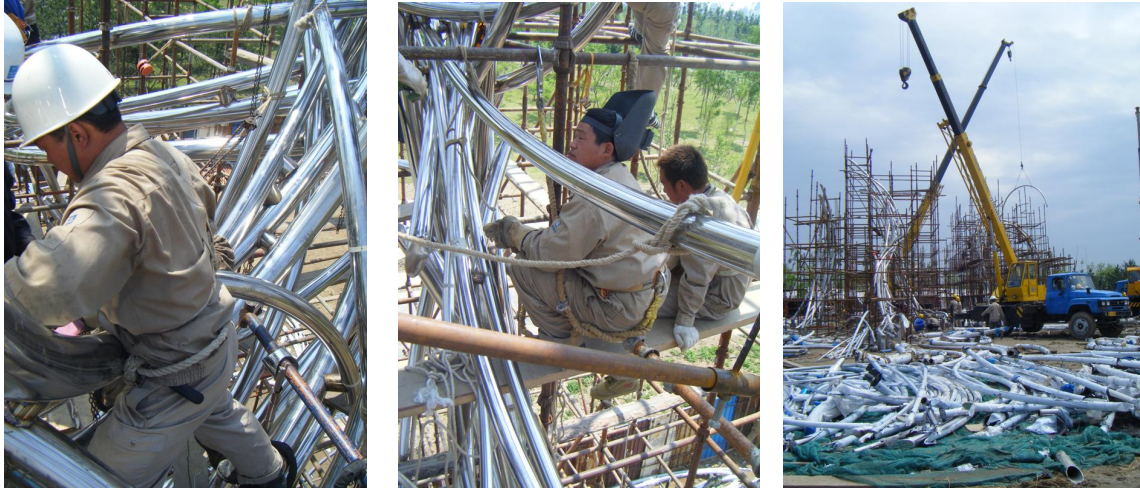
Fig.9: Construction process and on site assemblies
