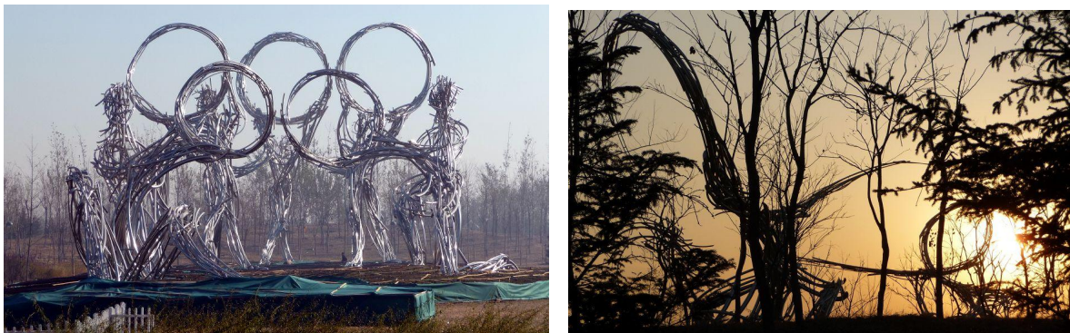
Fig.16: Final construction stage of the sculpture
