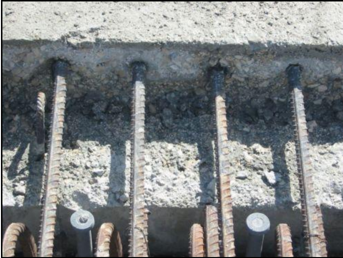
Figure 4.9: On site joint preparation
