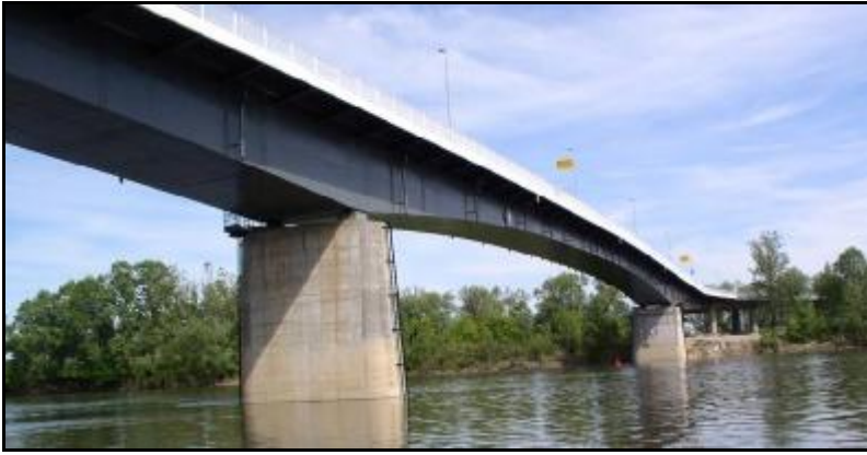
Figure 3.6: View of reconstructed main bridge across Sava River
