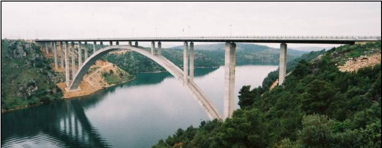
Figure 4.3: View of Krka River bridge
