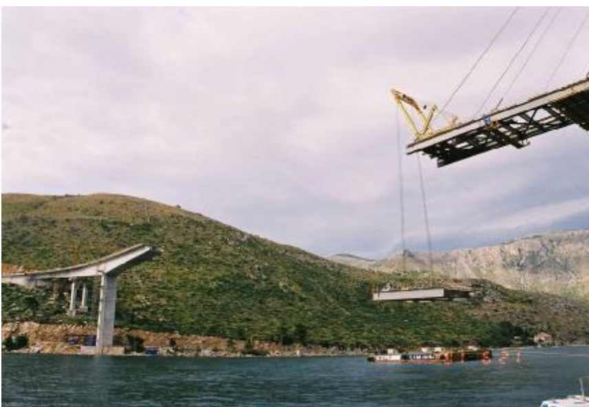
Figure 1.13: Lifting of one steel segment
