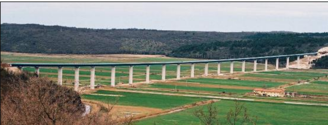
Figure 2.10: Some construction phases of Mirna viaduct
