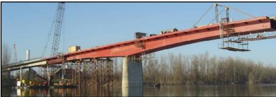
Figure 3.5: Free cantilever erection of new steel superstructure
