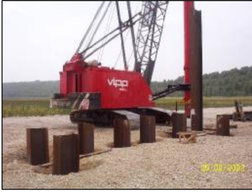
Figure 2.9: Construction of foundations
