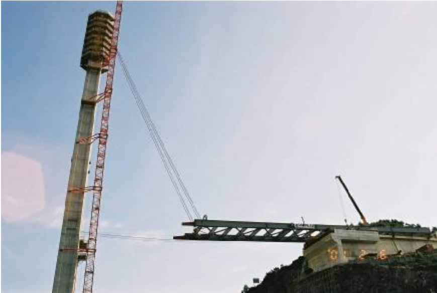
Figure 1.12: Launching of the steel grillage from east-end abutment
