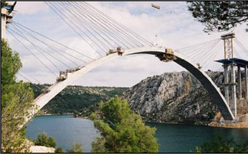
Figure 4.11: Arch closure segment construction of Krka River bridge
