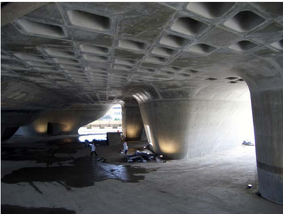
Figure 5 - ground level view at exposed wallfe slab
