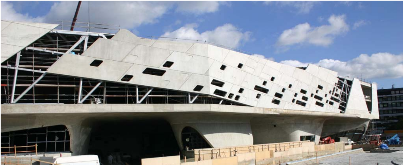
Figure 6 - south façade with pre-casted concrete panels
